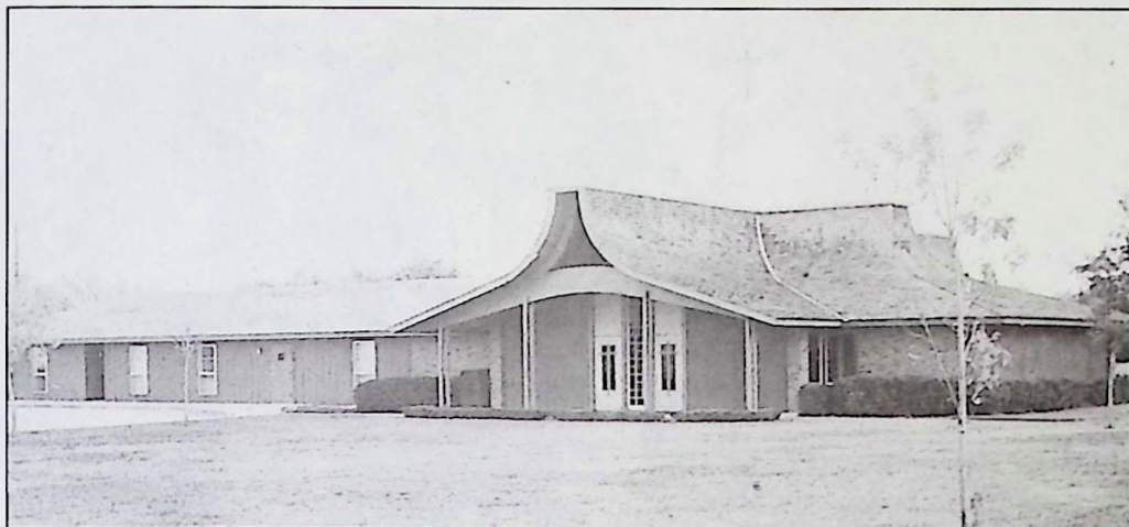
ASCENSION RISES —This new education and fellowship wing was dedicated Nov. 3 at Ascension Lutheran Church in Cleburne.
