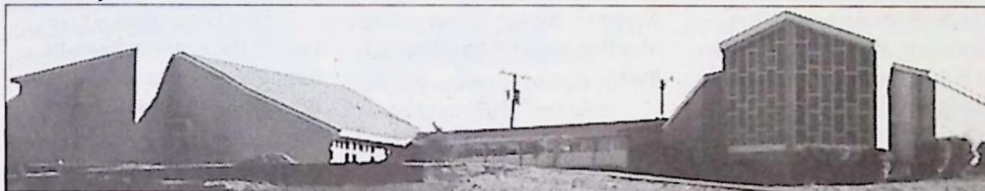
NEW LOOK —The skyline of Killeen was changed with the addition at Grace Lutheran of a new school building, left, and a renovated sanctuary. Grace sits at the entrance to Fort Hood.
