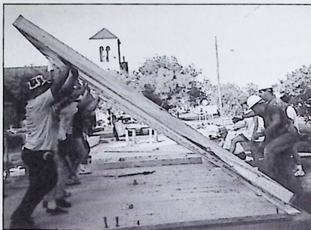
CAN-DOers raise the first wall of new church.
