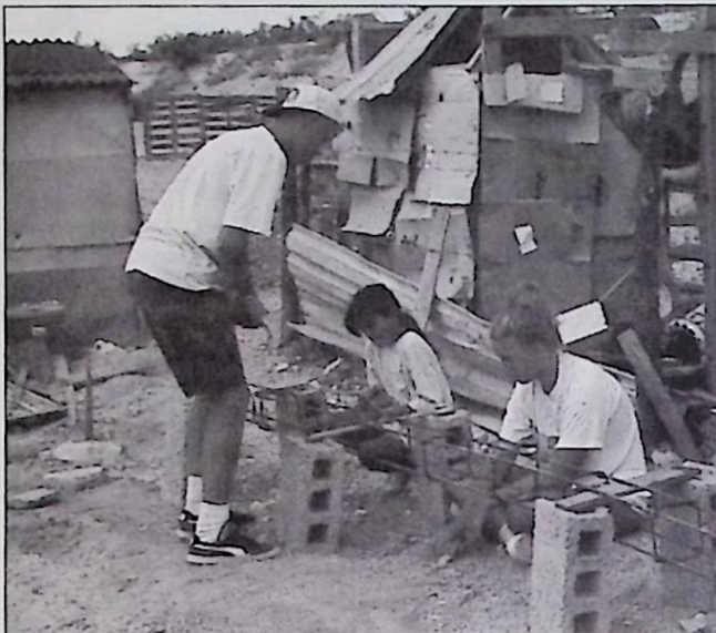
BUILDERS —CAN-DOers tie reinforcing steel as they help residents of Mexican colonia build houses to replace cardboard shacks like the one in the background.
