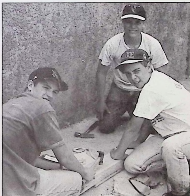
WOOD WORKERS —The only boys in the group from Memorial, Katy, work together on supports for the roof over the living quarters. They are, Brian Rice, left; Matt Hill, right; and Kendel Waggoner, rear. Photo by Lauren Rice.
