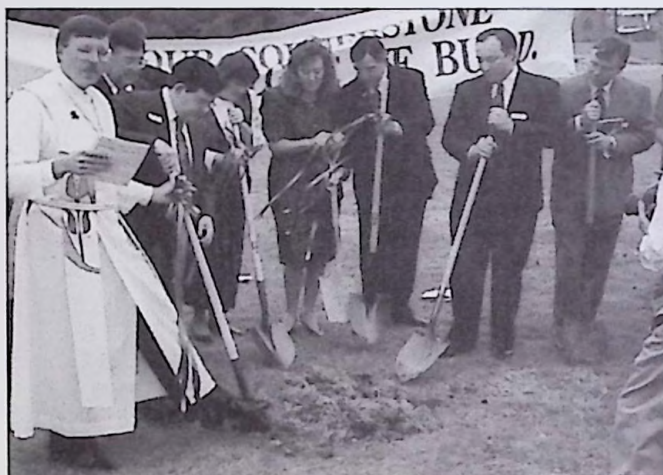
PLANO —Ground was broken at St. Paul, Plano, for a building expansion that will include Sunday school rooms, larger fellowship hall, nursery improvements and office space. John Kah is senior pastor.
