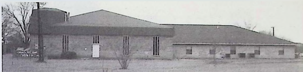
ADDITION —This is Christ the King Lutheran in Waxahachie with its new educational wing.
