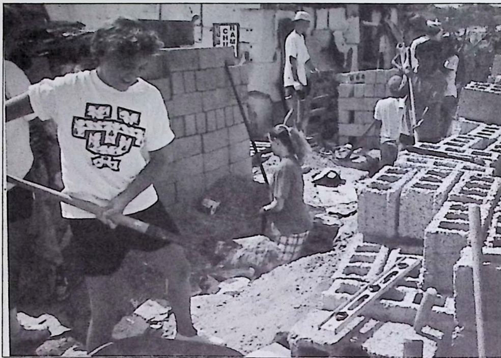
SERVANTS —Project CAN-DO youth and adults will build a house in Del Rio this summer.
