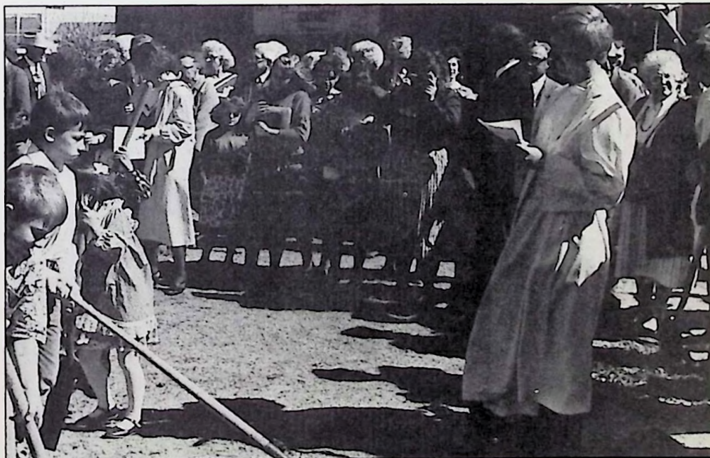
VERNON —Rev. Rusty Leavitt, right, and children of St. Paul Lutheran Church, Vernon, take part Feb. 25 in groundbreaking for an activities and classroom building. The structure will include a gymnasium, four pre-k-
