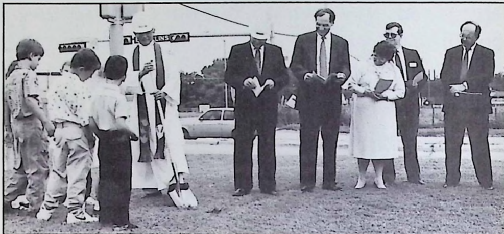
EXTENSION —Concordia Lutheran of Garland broke ground June 3 for extension of its present multi-purpose building. That's Senior Pastor Gerald Nichols with the shovel. The extension will add 8,500 square feet and include 18 new classrooms and three administrative offices. Building plans include enlarging the narthex, nursery and parking lot. Total program is about $400,000. Future plans include a large sanctuary in the next three to five years.
