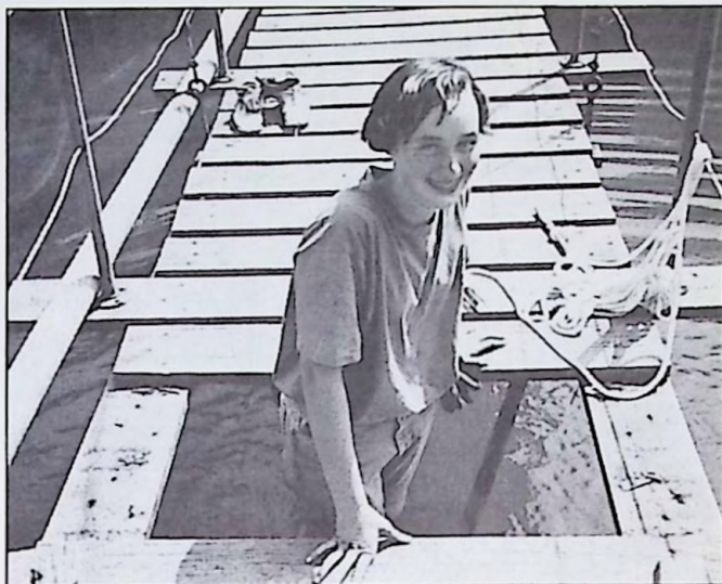
COLD FEET —Staying cool while repairing a suspension bridge damaged during spring flooding at Texoma Lutheran Camp is this member of a Servant Event team.
