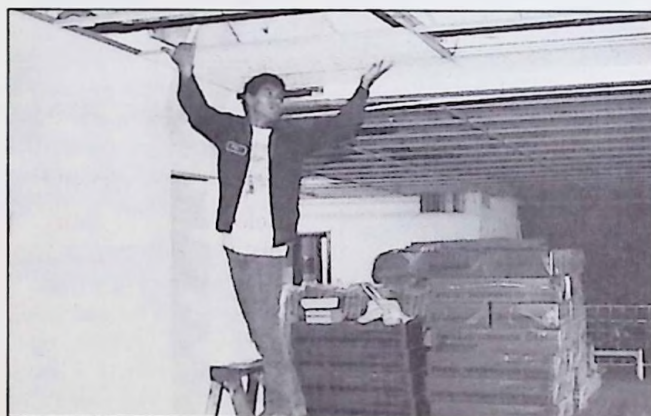
REMODELED —A workman installed ceiling tile in Bethesda's new Austin thrift store. Volunteers did much of the painting.
