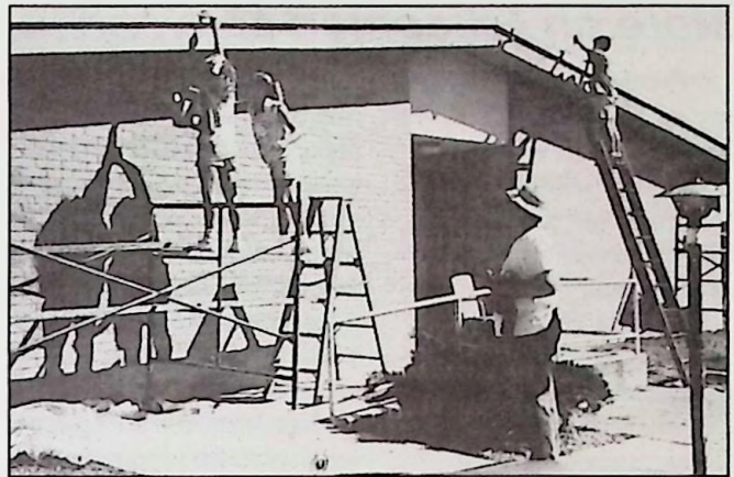
ON A MISSION —Members of the junior confirmation class of Holy Comforter Lutheran Church of Houston paint a building at Trinity Lutheran Home in Shiner.
